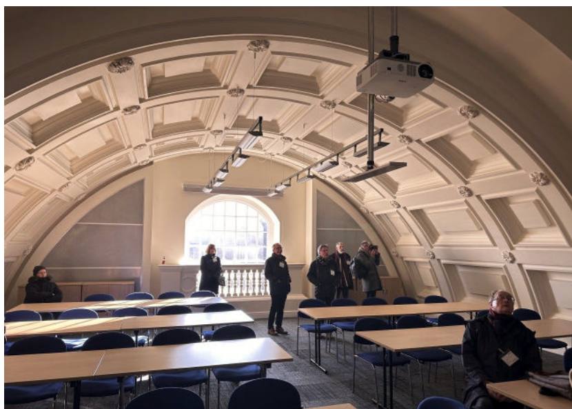
The coffered, barrel-vaulted ceiling in the Great Hall at BMA House. Photo © Paul Waite
